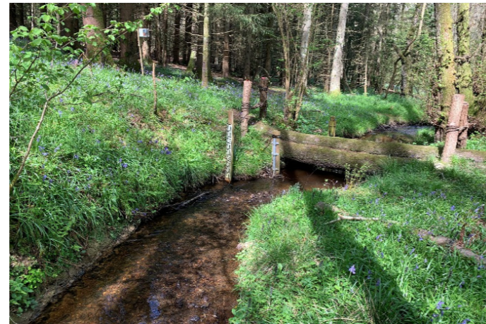
Figure 3 Example of a Leaky Dam in the Surrey Hills
